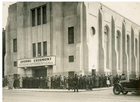
Re-opening of Poplar Methodist Church following major renovation work, 30th September 1933
