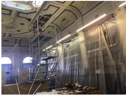
A scaffold tower has been erected to facilitate investigations of the damage to the ceiling. Shelving has been sheeted off to protect books from dust.
